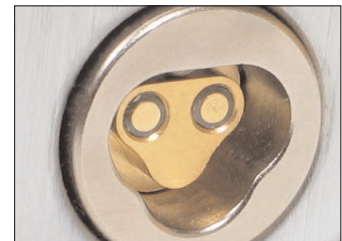
Figure 3: Gold-plating on lock face with two contact points
